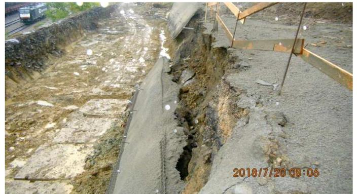
Figure 13. Crack zone
