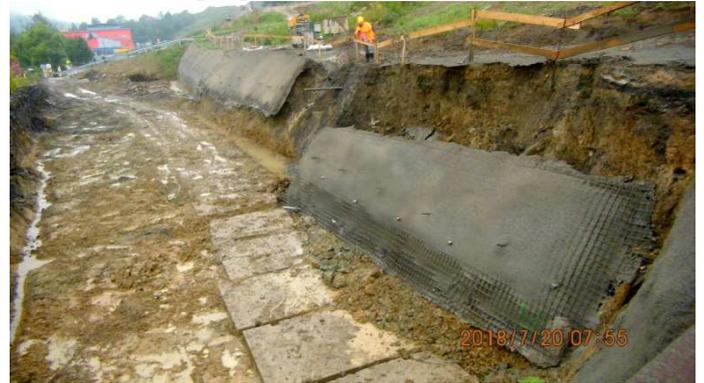
Figure 12. More than a week open unsecured excavation and one-day rain
